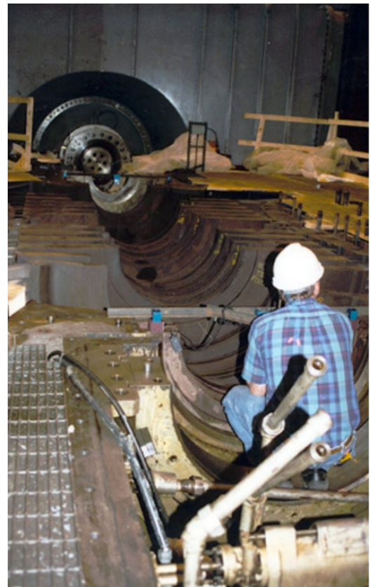
Aligning Steam Turbine Diaphragms with L-706
